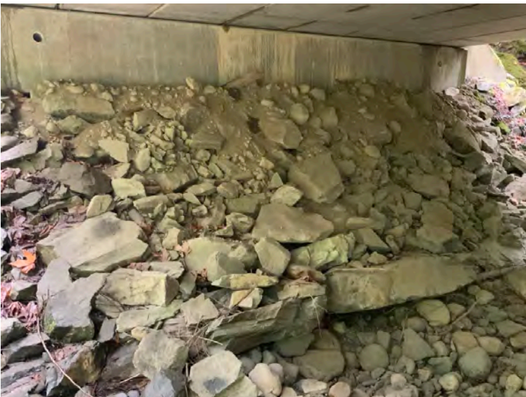
Left Bank Abutment when facing downstream
