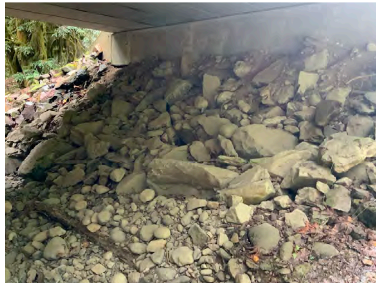
Right Bank Abutment when facing downstream
